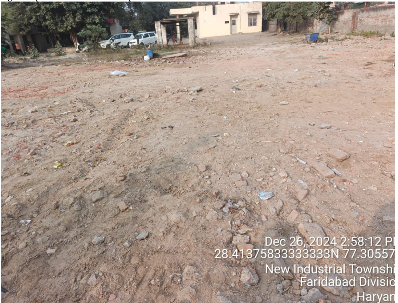
Fig 4 leveling of area with soil after cutting of trees
